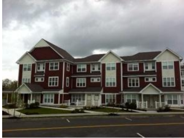
Construction at Olmsted Green
