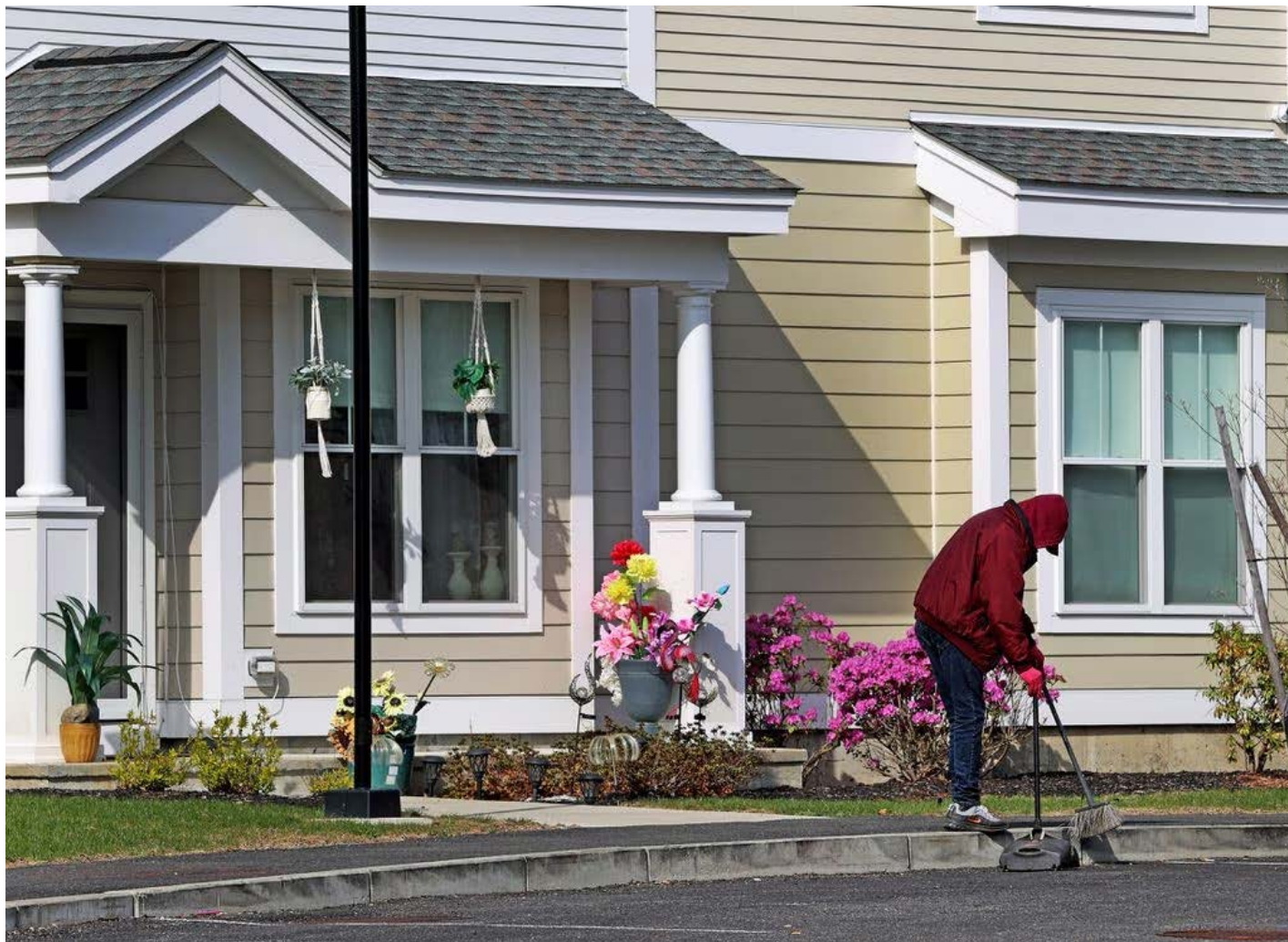
Built on the site of an old Mattapan mental hospital, Olmsted Green is a neighborhood of nearly 1,500 people in single-family homes and apartments, along with two charter schools and a new community center. DAVID L. RYAN/GLOBE STAFF
